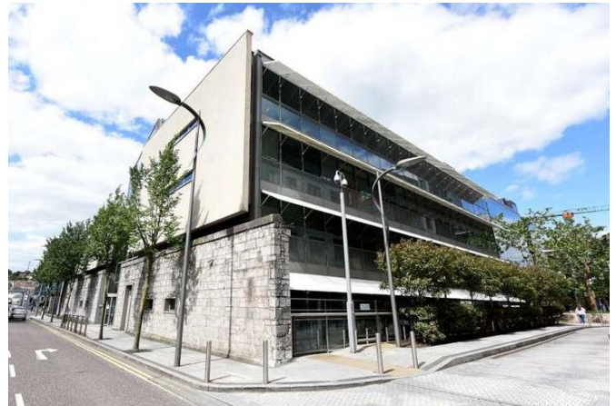
Office property in Cork, Ireland
