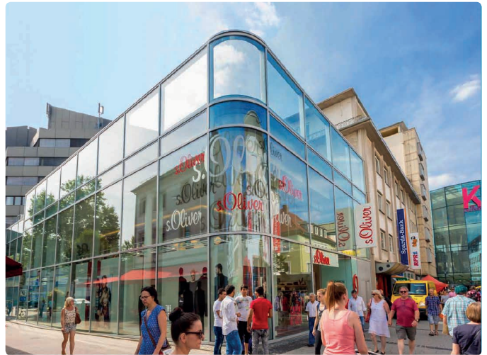
Fackelcenter Shopping Centre, Kaiserslautern
