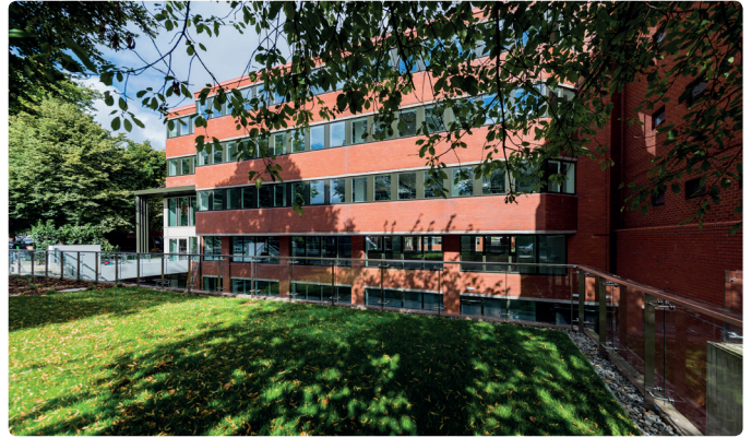
Two Haddington Buildings, Dublin (VSREE)
